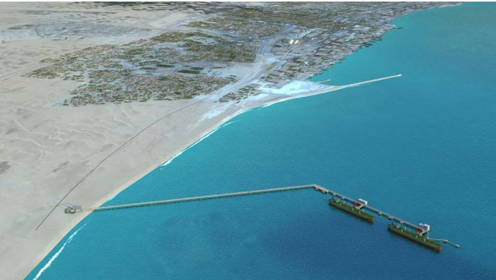
National Oil Storage Facilities – Walvis Bay, Namíbia
