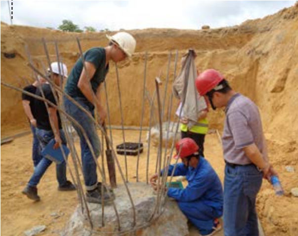
PILE TRIMMING
