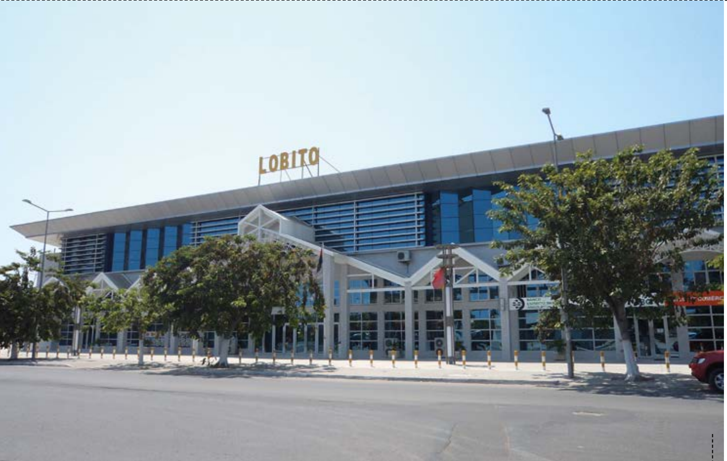
MAIN FRONT OF THE LOBITO STATION
