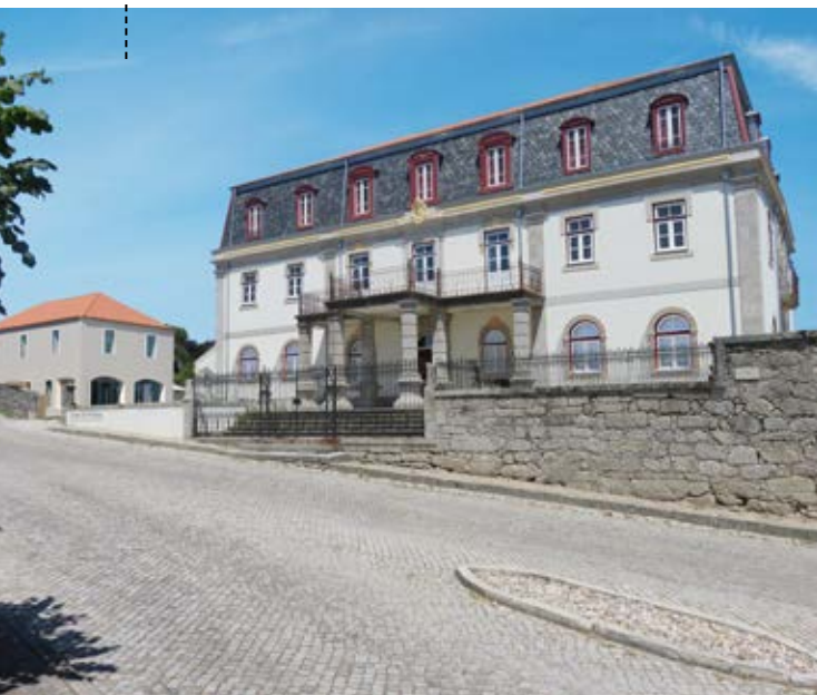
VIEW OF THE MAIN ENTRANCE
