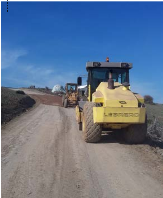
START OF THE REHABILITATION WORK
