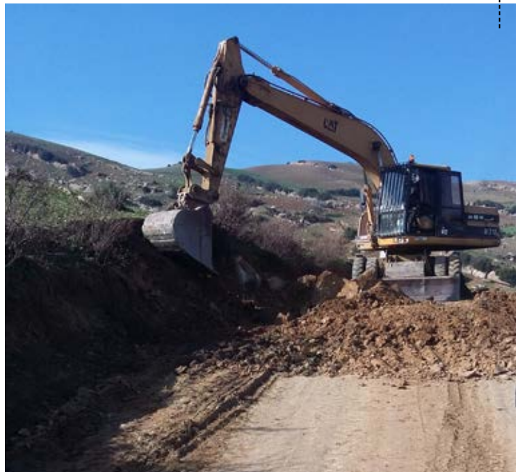
START OF THE REHABILITATION WORK
