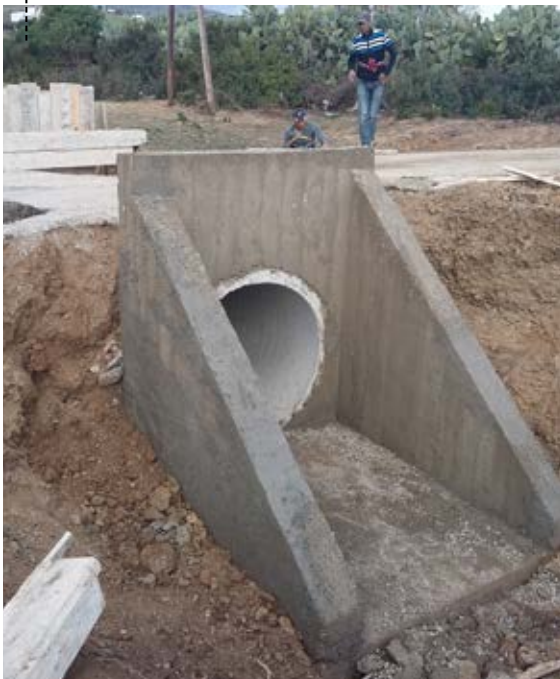
VIEW OF A CULVERT
