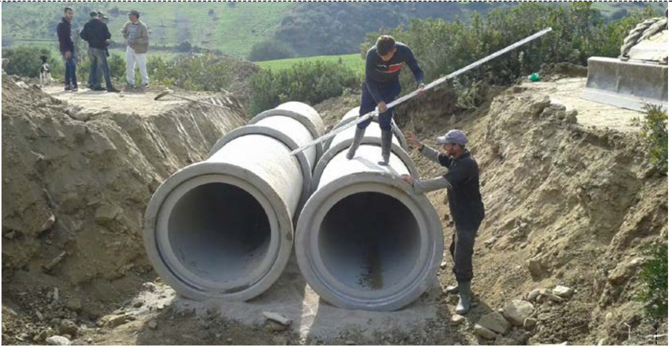
CULVERT INSTALLATION
