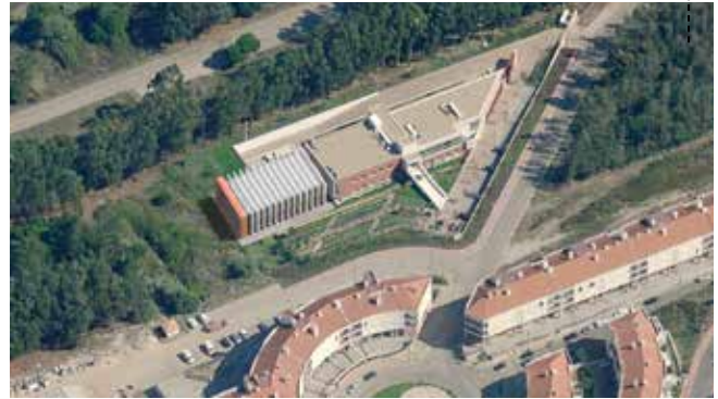
AERIAL VIEW – AFTER
