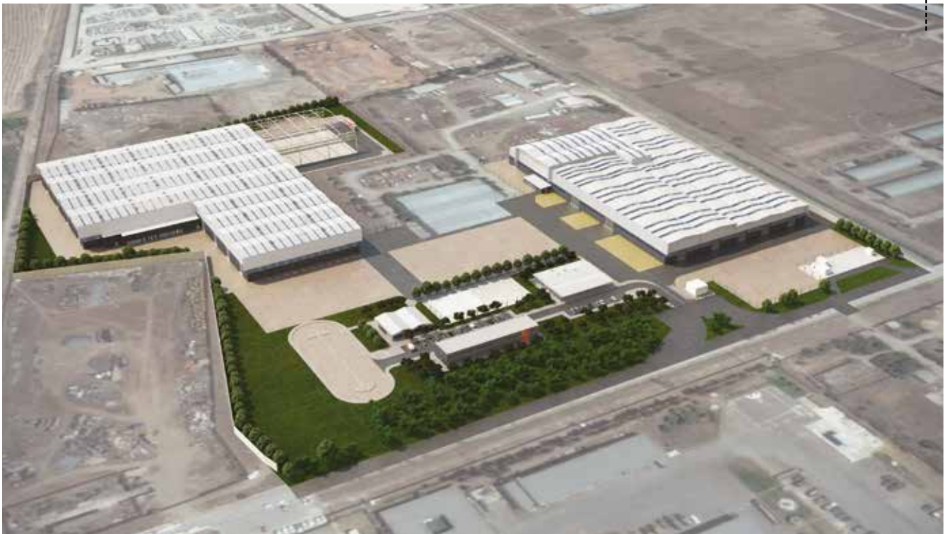
OVERVIEW OF THE COMPLEX
