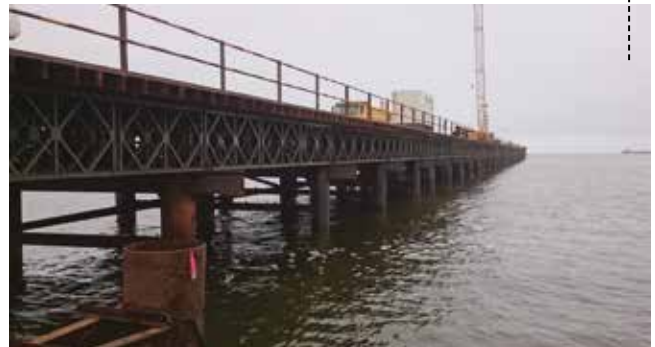
TRESTLE AND OIL TANKER JETTY CONSTRUCTION WORKS
