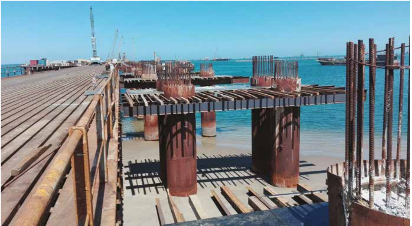
TRESTLE AND OIL TANKER JETTY CONSTRUCTION WORKS
