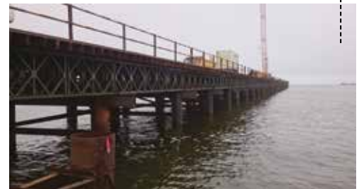
TRESTLE AND OIL TANKER JETTY CONSTRUCTION WORKS
