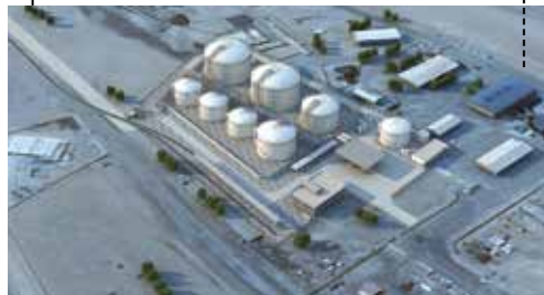
AERIAL VIEW OF THE TANK FARM
