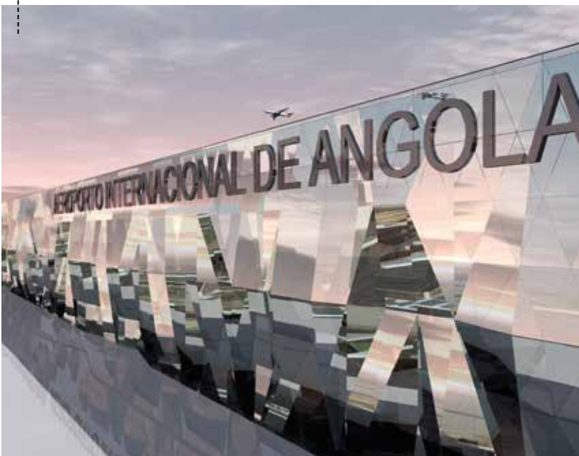
MAIN FRONT OF THE PASSENGER TERMINAL
