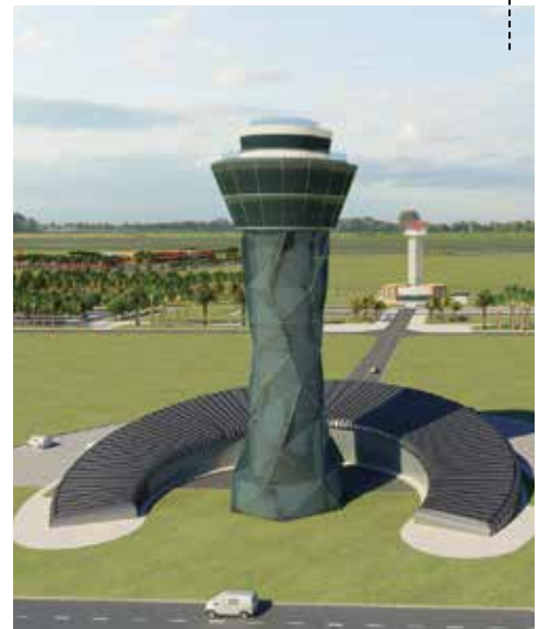
CONTROL TOWER AND TECHNICAL BLOCK
