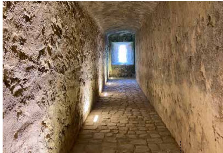
VIEW ON INTERVENTIONED PASSAGE
