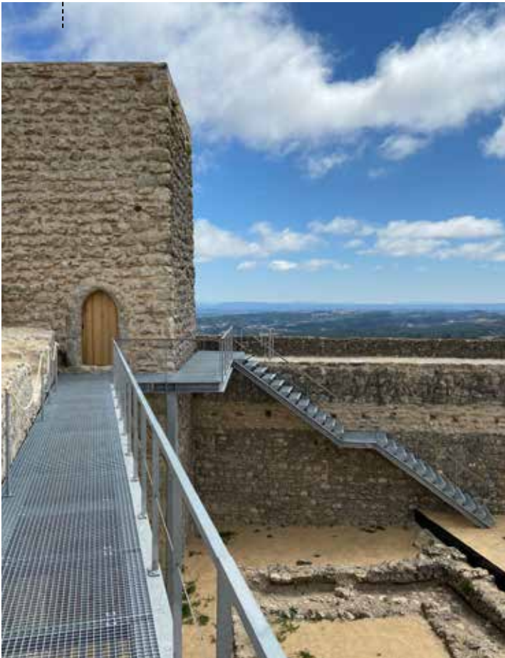
WALKWAY CONNECTION AND STAIRS
