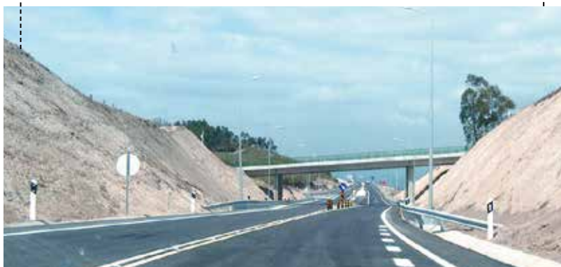
OVERPASS NEAR LAMEIRÃO
