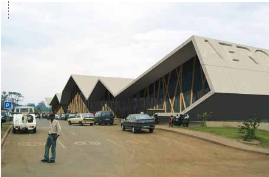
TERMINAL MAIN ACCESS
