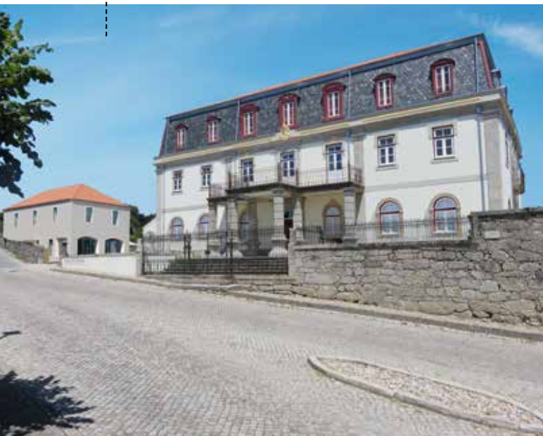
VIEW OF THE MAIN ENTRANCE
