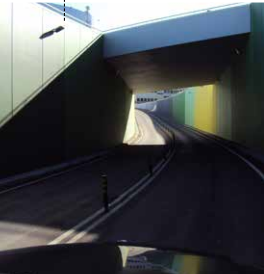
VIEW OF THE ROAD UNDERPASS
