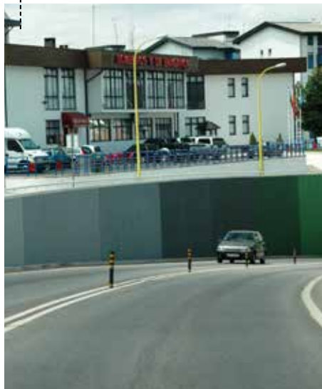
BEGINNING OF THE GRADE SEPARATION
