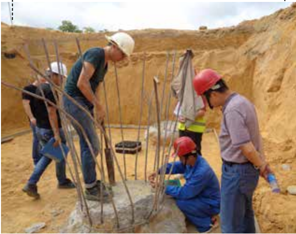
PILE TRIMMING
