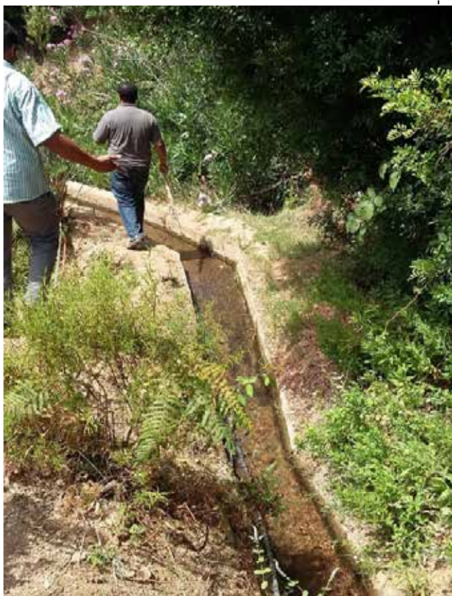
DIAGNOSIS OF AN EXISTING IRRIGATION CANAL
