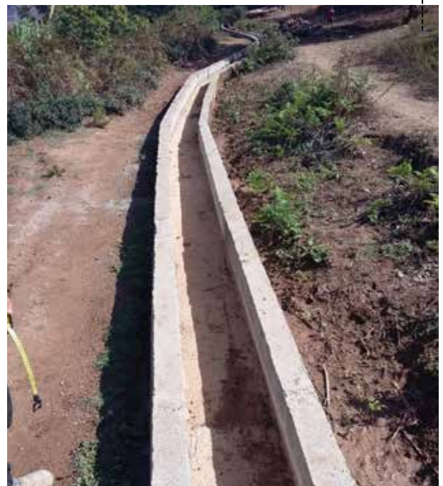
FINAL IRRIGATION CANAL
