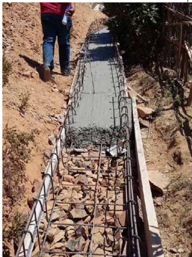
CONSTRUCTION OF AN IRRIGATION CANAL
