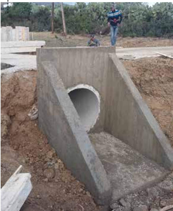
VIEW OF A CULVERT
