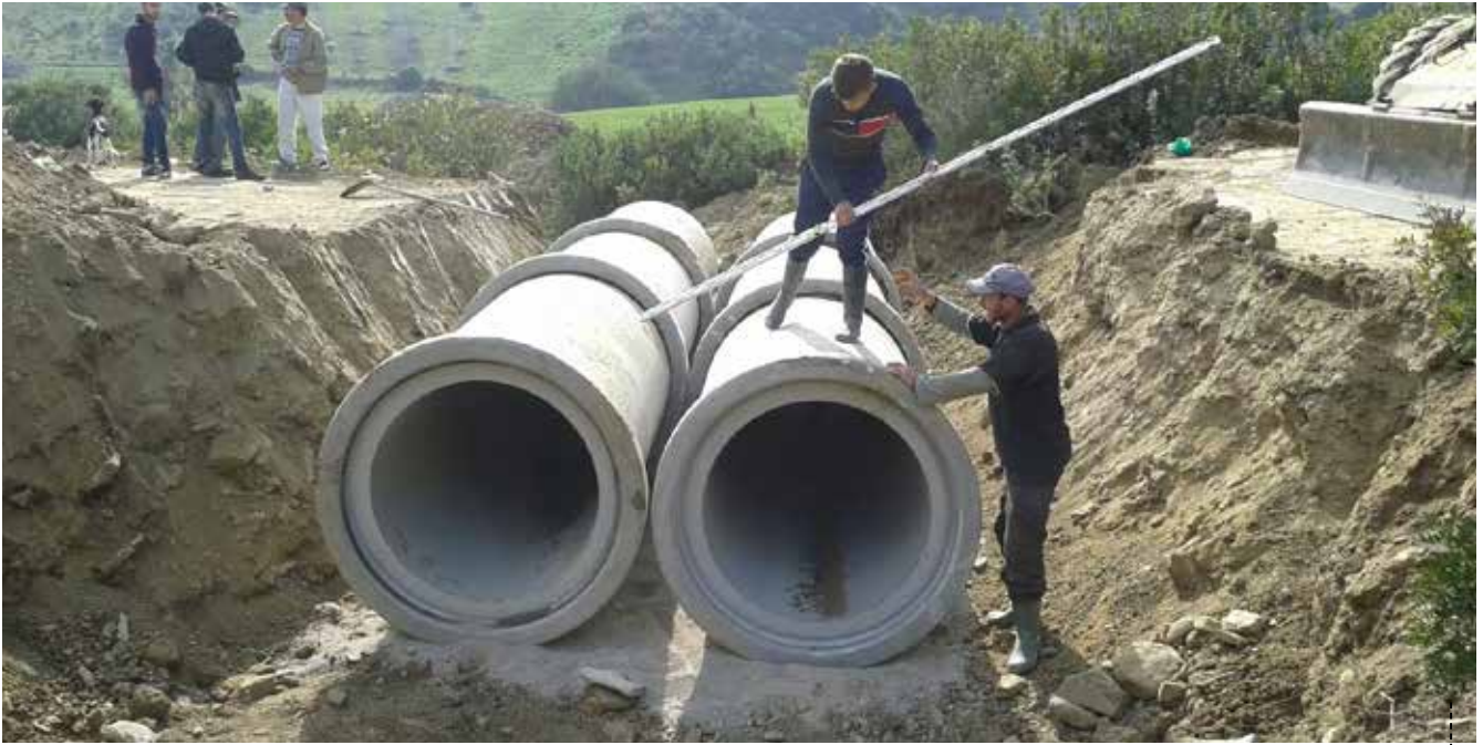
CULVERT INSTALLATION
