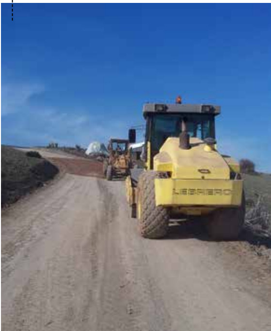
START OF THE REHABILITATION WORK
