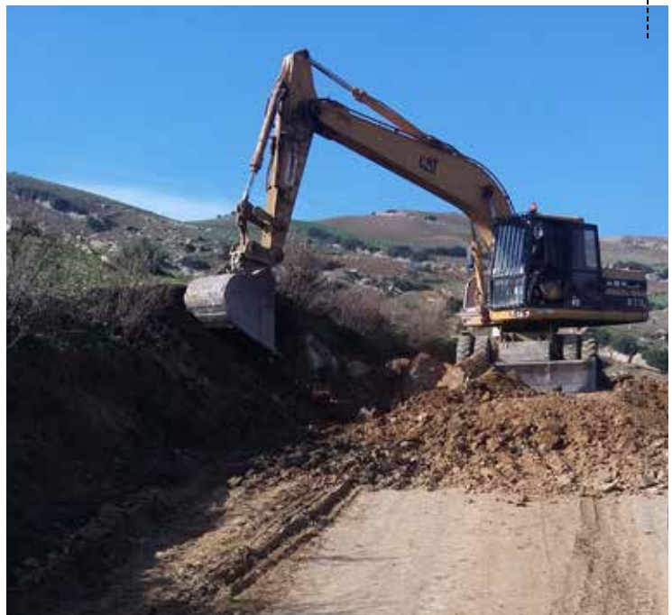
START OF THE REHABILITATION WORK
