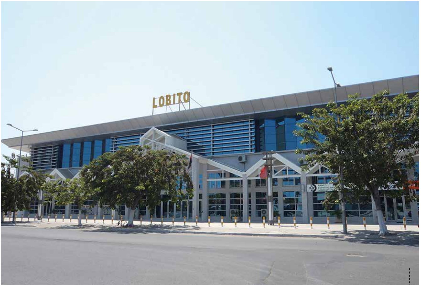
MAIN FRONT OF THE LOBITO STATION
